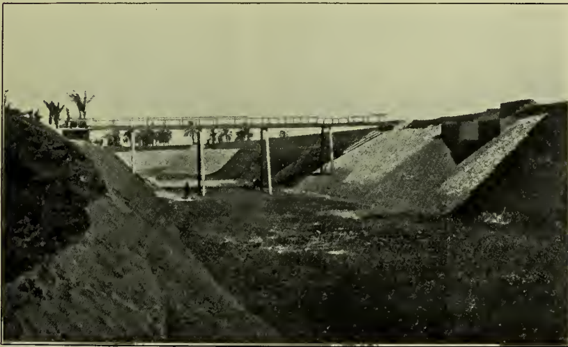
Road Bridge, Kilibia Canal.
