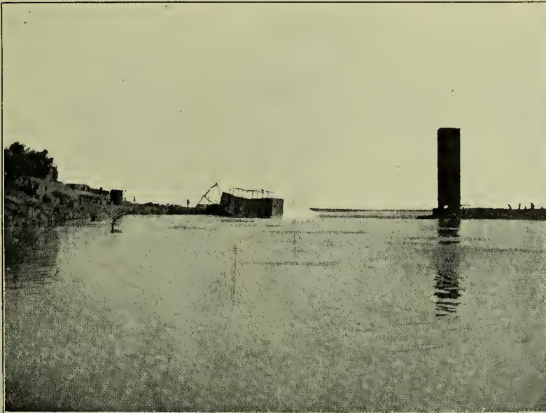
Closing the old Hindia Barrage Breach (from Upstream).
