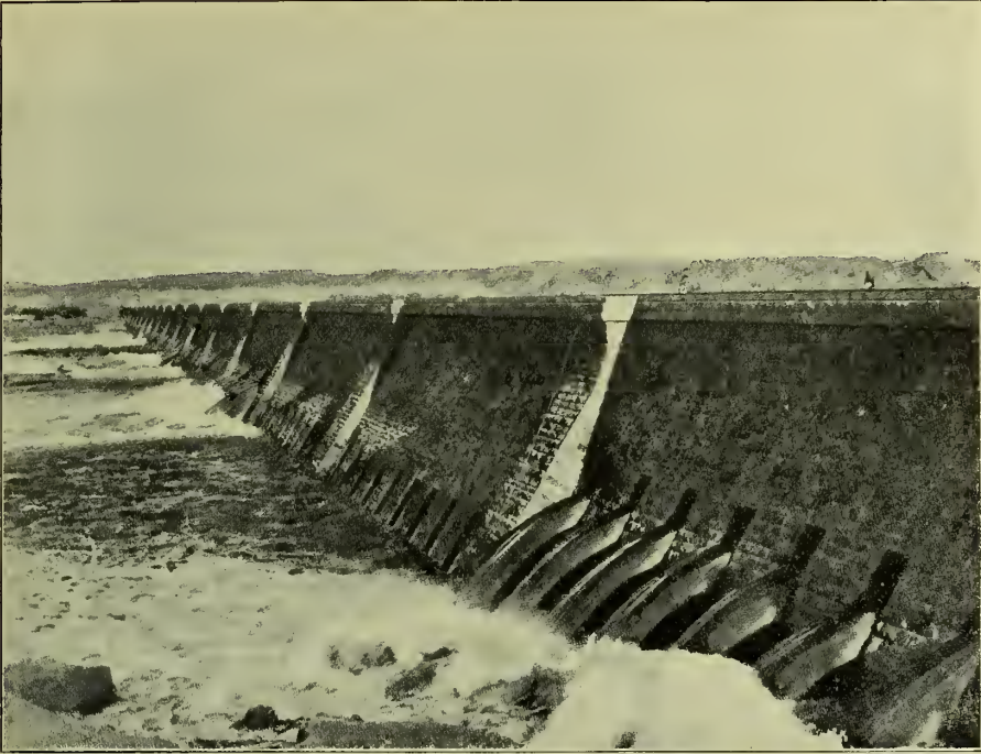
The Aswan Dam before the Construction of the Talus.
